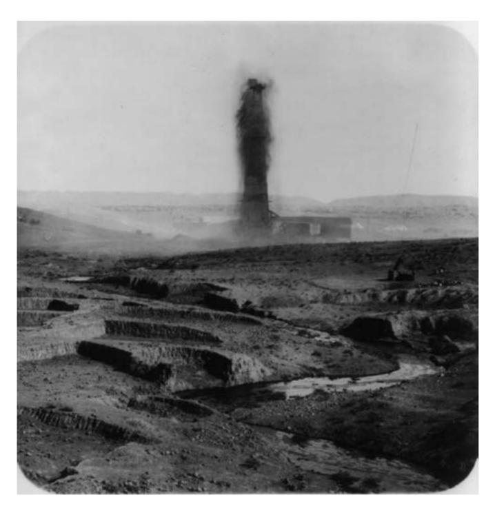
on the forces of nature. Natural water or gas, reacting to pressure differences in underground basins, is generally what pushed the oil to the surface. Initially, this often occurred with great force, as we know from the famous images of blowouts or 'geysers'.
